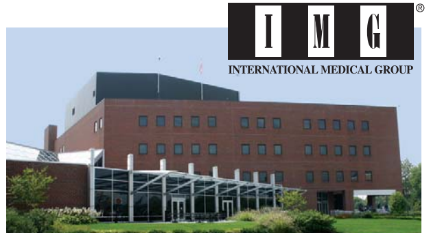
IMG World Headquarters, Indianapolis, Indiana
